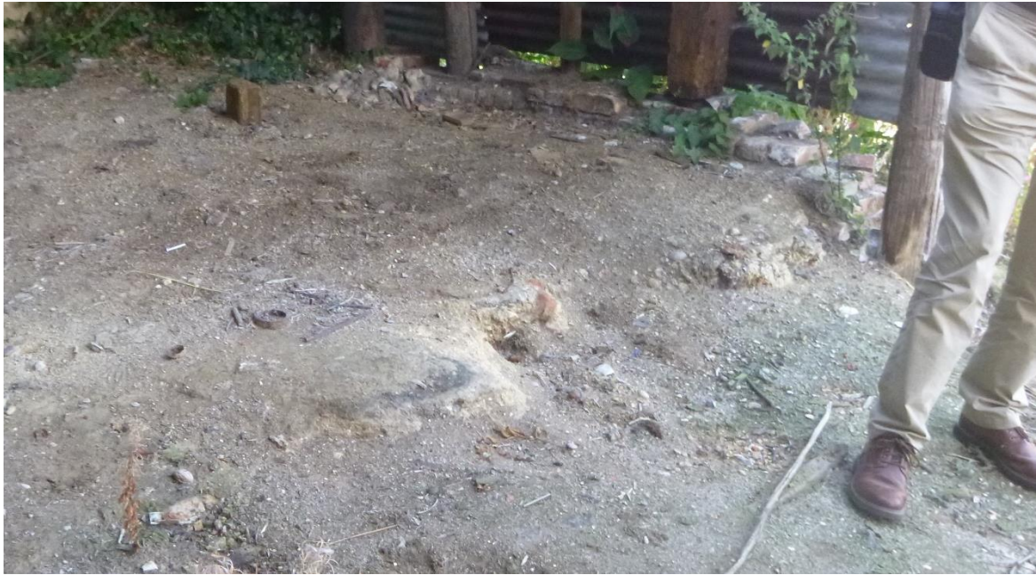
The probable remains of clay internal flooring, perhaps original to the house
